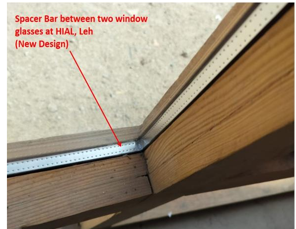
Double Glazed Wooden Window with Spacer Bar
