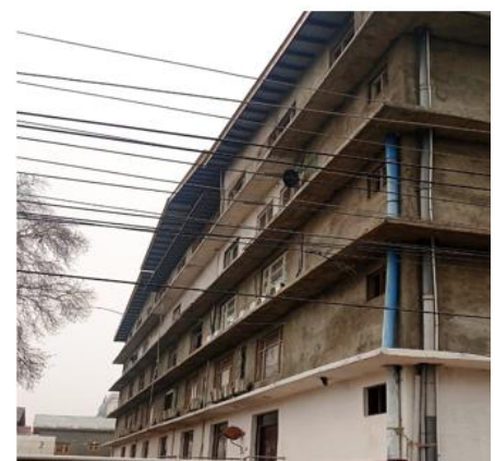
Window shades, verandas, balconies, cause of heat loss during winter and heat gain during summer
