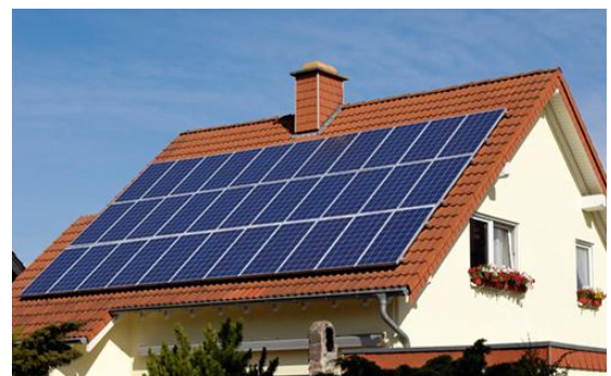
Simple Roof favourable for Solar Modules, insulation and maintenance
