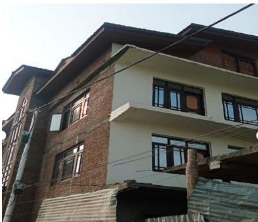
Window shades, verandas, balconies, cause of heat loss during winter and heat gain during summer
